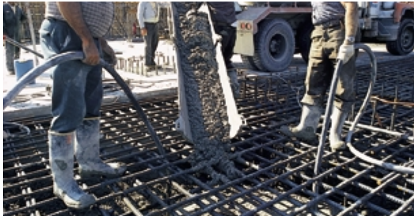
Figure 4.18 Reinforced concrete can withstand both tension and compression. It is used to make buildings, bridges, and other large, strong structures.
